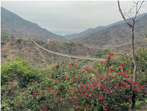
We visited the Jorullo Bridge across the Cuale River outside of town, 500 feet over the stream; about 1500 feet from end to end.
