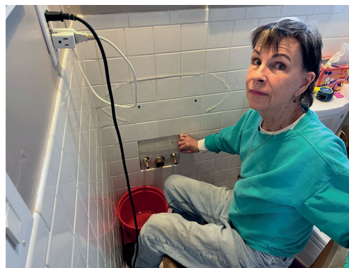
Preparing to mount the tiles.
